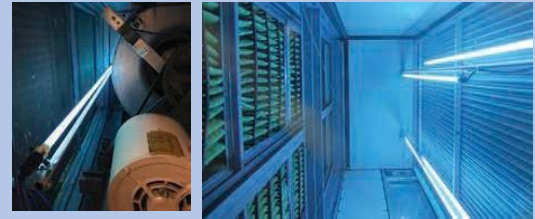
UV-C light keeps coils free of mold
